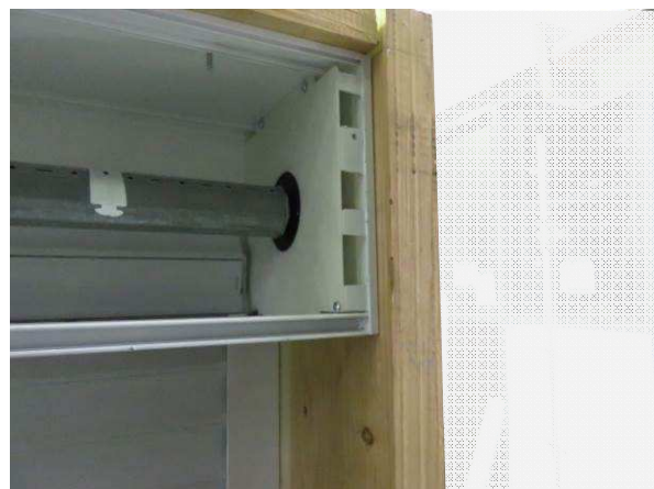
Figure 8 Roller shutter box - rear opened
