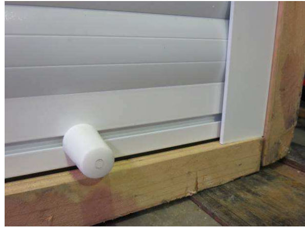
Figure 4 Bottom lath and guide rail
