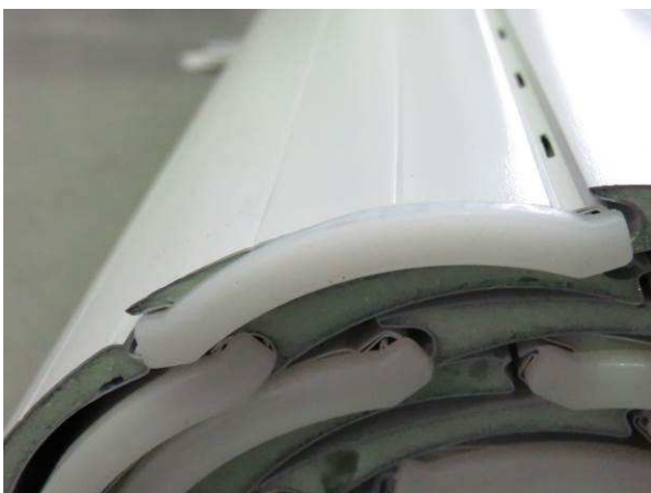
Figure 7 Details of lath profile with slider
