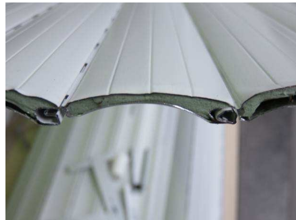
Figure 6 Details of lath profile
