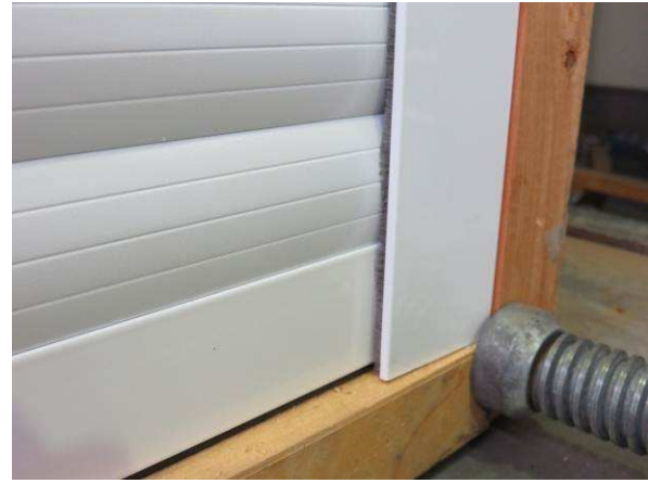
Figure 4 Bottom lath and guide rail
