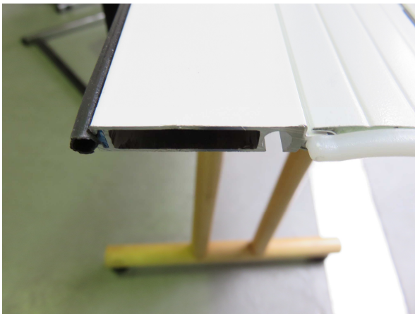
Figure 5 Detail bottom lath
